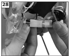
Connect plug from fan to switch house plug.
